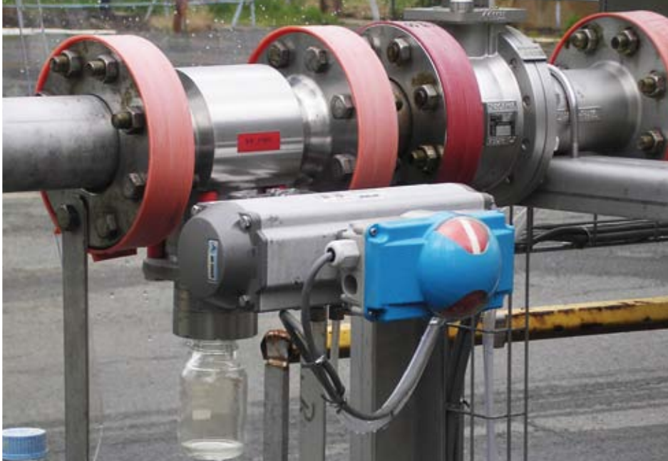
Sampling of acid for quality control
