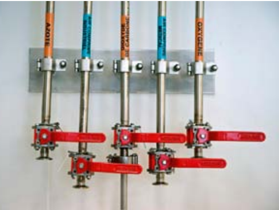
Valves with welded and clamp connections in a research laboratory
